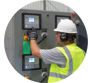
System enhancements and integrity work
